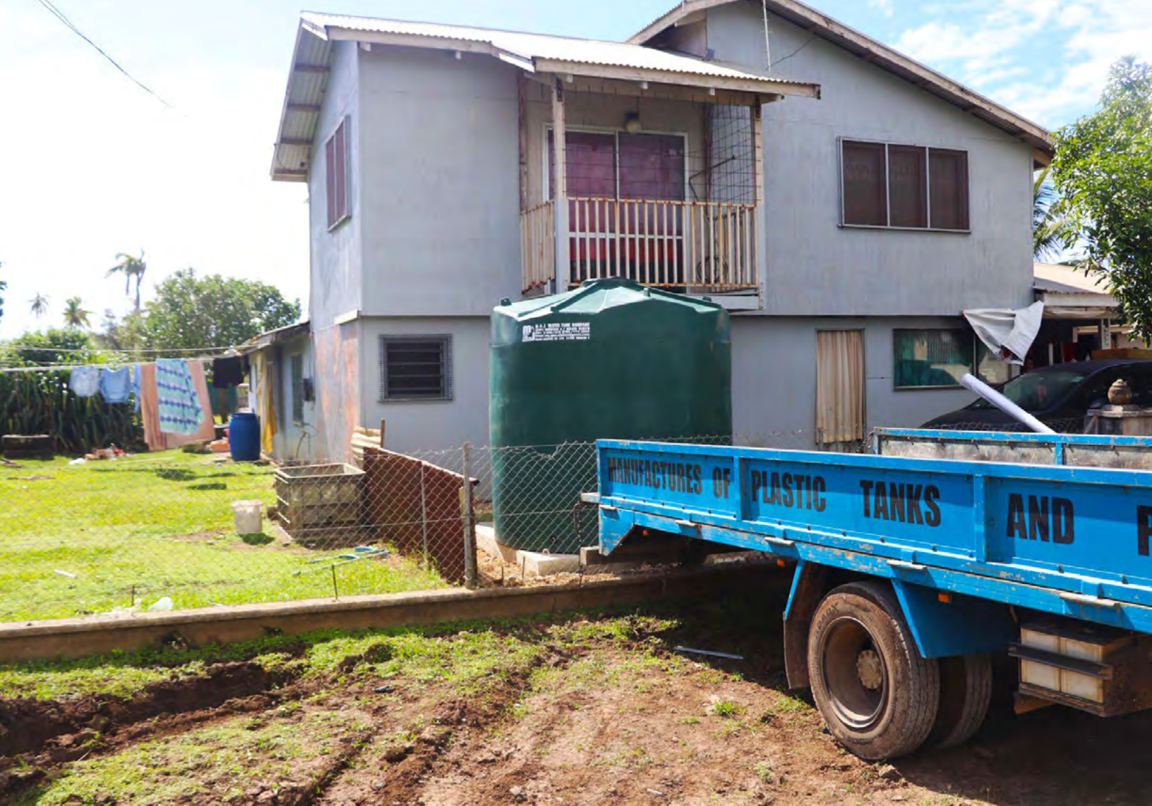
▲ The National Water Tank Project is currently underway on the main island of Tongatapu. (Viliani Takau)
