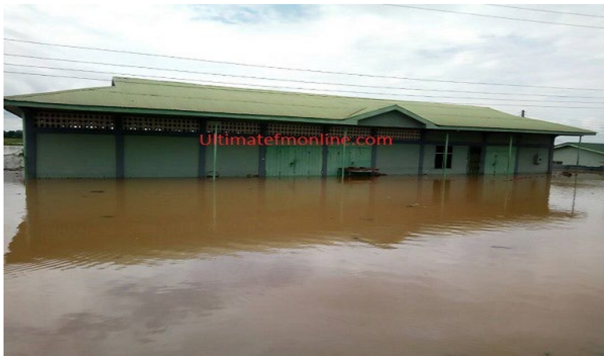
Photo of a flooded facility as result of the collapse of the River Odo bridge in 2017.
