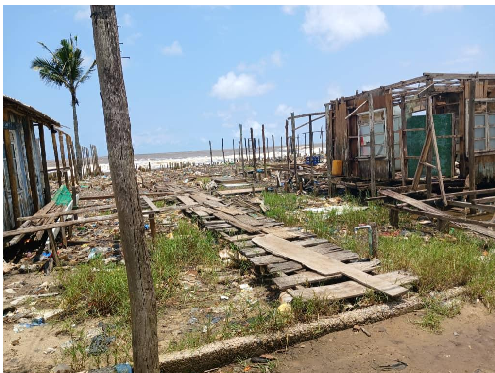
Figure 5. Devastation caused by sea surges in Ayetoro
